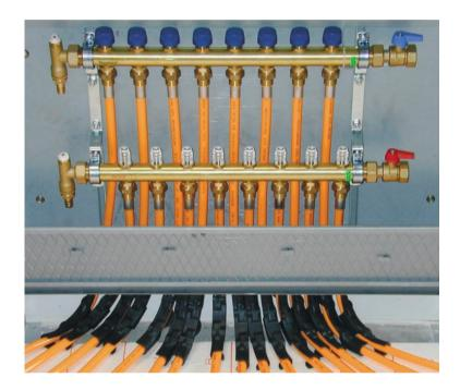
The manifold station for radiator connection contains  $\frac{3}{4}$ " euro-cone outputs that can be connected by pressing or clamping using coupling adapters.
